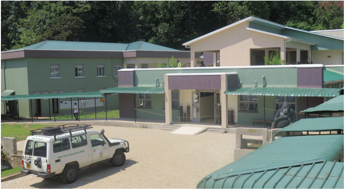
The completed medical ward
