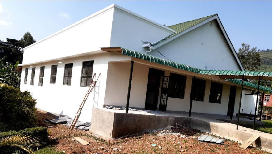
Expansion of the dining hall at UNSB
